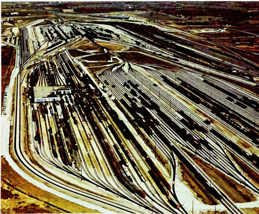
At Canadian National's yard in Vaughan Township, 5,000 cars are marshalled by computer, radio, radar, teletype and old-fashioned gravity, in the world's most advanced freight-handling facilities.
