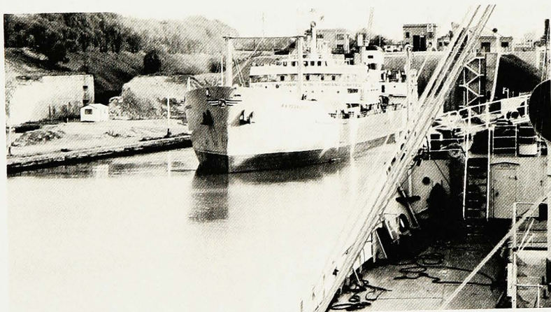
Part of the world's biggest seaway, the 26-mile Welland Canal passes ocean-going ships between lakes Erie and Ontario—a fall of 327 feet.
